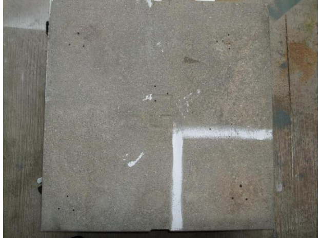
(b) After removal of Coating
